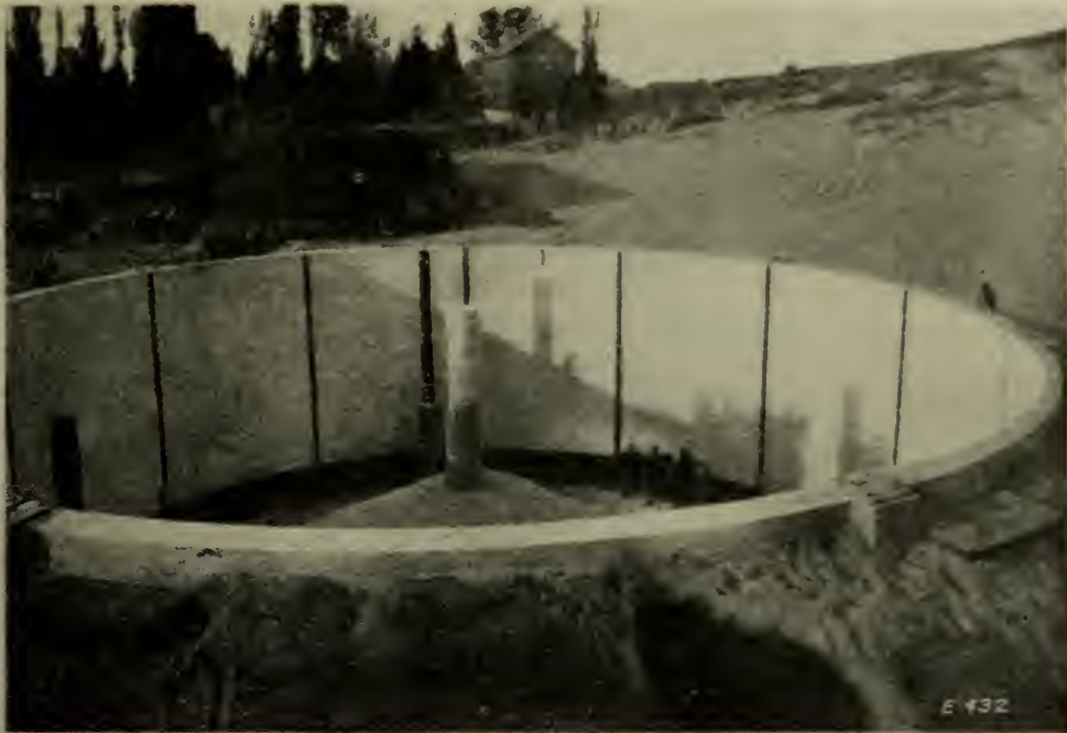
FIG. 4. CONCRETE GAS HOLDER TANK.
